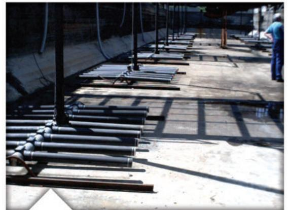
These liftable fine bubble tube grids on guide rails have worked over 10 years in this municipal WWTP
